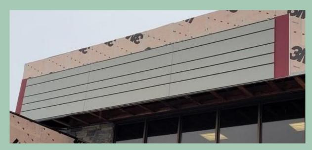
The Proclad Aline Series is a true pressure equalized rain screen system. The vented air space behind the panel face keeps the cavity dry resulting in long term performance.
